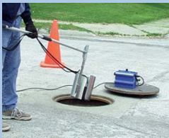
Isco Street Level Installation Tool
